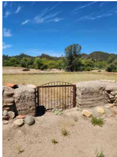
Donnie Pierce Jr. Placed the Adobe blocks on the right side of the gate. The gate was built by Matthew Briggs.
